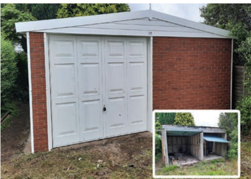
Hanson Garage Refurbs Pages 28-29
